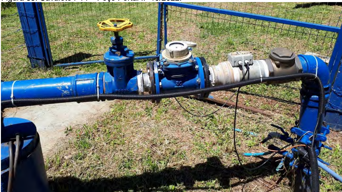
Figura 85: Cavalete P14 – Poço Portal II -10/2022.
