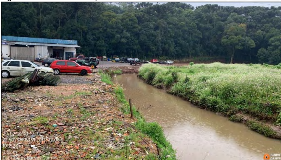
Figura 329: Arroio do Hospital – 09/2022.
